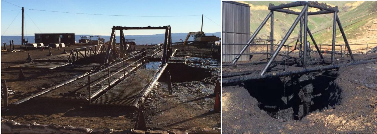
Figure 8. Vent crater caused by expulsion of top kill attempt materials
