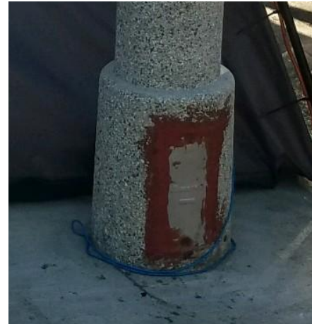
Seal Handholes and Pullboxes with Epoxy
